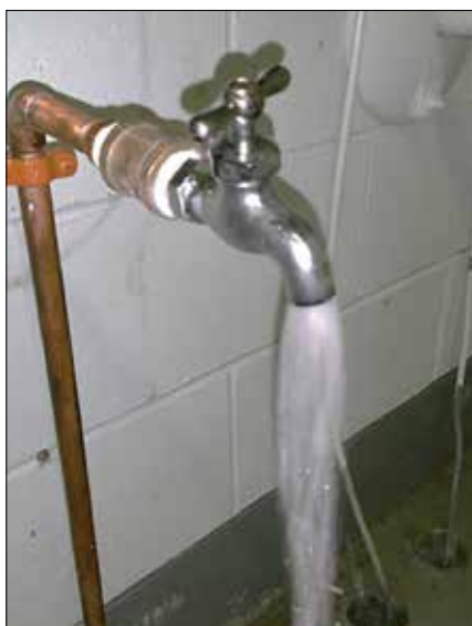
Figure 1 - Smooth-nosed sample tap
