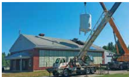
Installation of the GAC filters September 2016.
