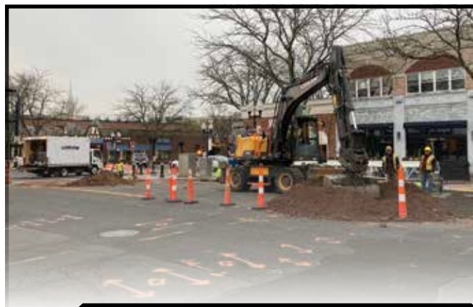
The Metropolitan District installing a 24-inch water main.
