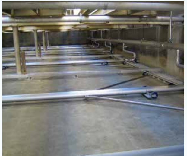
MRI HOSELESS CABLE-VAC SLUDGE COLLECTOR
