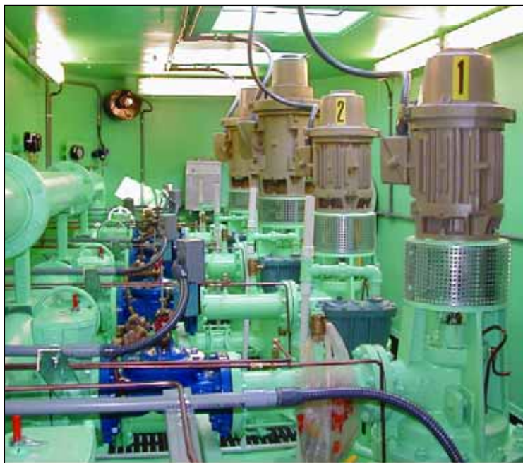
(Above) EFL factory built pump station, installed and operational in a fraction of the time it takes to build a pump station on site.
