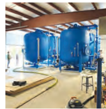
Mill Road PFAS WTP during construction.
